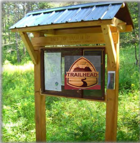
NEW INFORMATION SIGN WITH GREEN METAL ROOF AND RECLAIMED 8x8 WOOD POSTS
